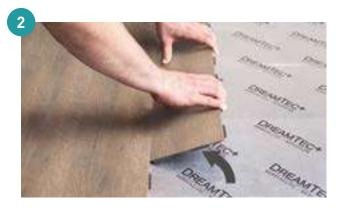
To complete the joint, lift the outer edge of one plank upwards to approximately 20°. You don't need to use a hammer to put the planks together.
