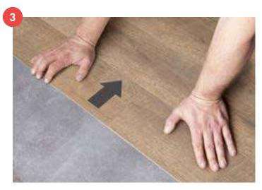
Gently push the entire plank down. Pull the long side of the plank towards the previously installed row to ensure a perfectly tight joint. Press the planks to ensure good adhesion to the subfloor.
