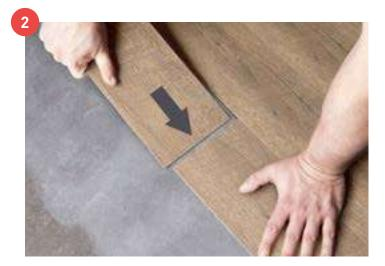
Push the short edges of the planks together whilst holding the already installed plank in place.
