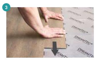
Gently push the planks together to achieve a perfectly tight joint, then lock the joint by lowering the plank back flat onto the floor.
