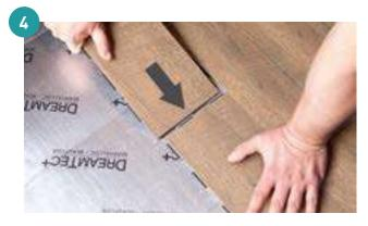
Thanks to the four-sided click system, you can lock the planks along either the long or short sides.
