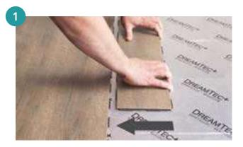
Join the planks by positioning and sliding them towards each other flush with the floor so that the connector tabs start to interlock.
