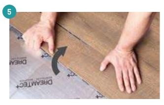
Join the short side so that the connector tabs start to interlock. Slide the long side into the previously installed row. Lift slightly, click and push down.
